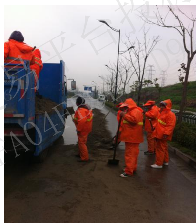
再将渣土装入自卸车清运车
